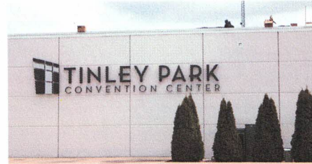
The 75,000-square-foot Tinley Park Convention Center is being considered by the U.S. Army Corps of Engineers to house COVID-19 patients as a way to ease the burden on local hospitals. Photo credit: Wendell Hutson
